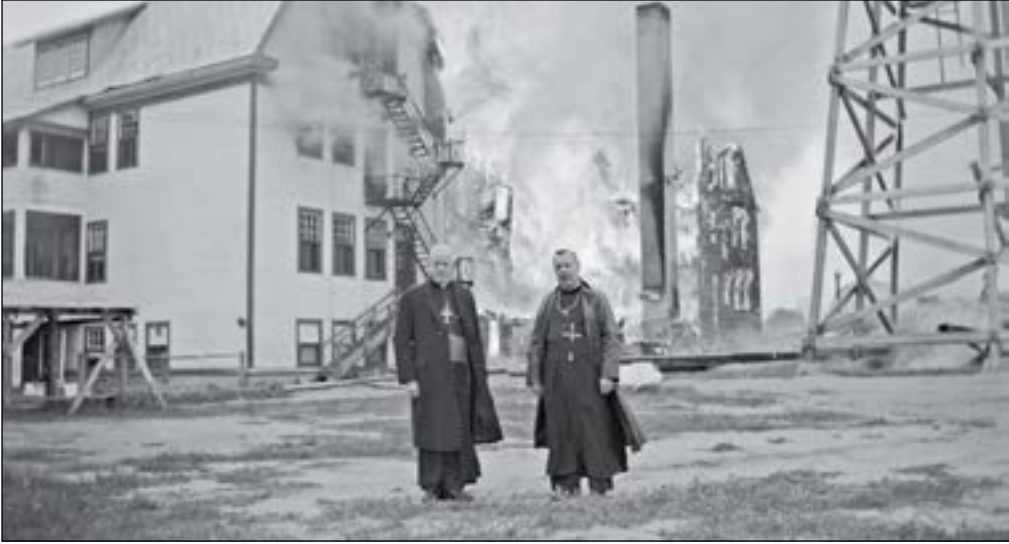
The Roman Catholic school at Sturgeon Landing, Saskatchewan, was destroyed by fire in September 1952. There was no loss of life. St. Boniface Historical Society Archives, Roman Catholic Archbishop of Keewatin-The Pas Fonds, N3637.
