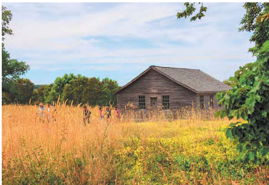
Former mission site at Lake Condah, February 2023
